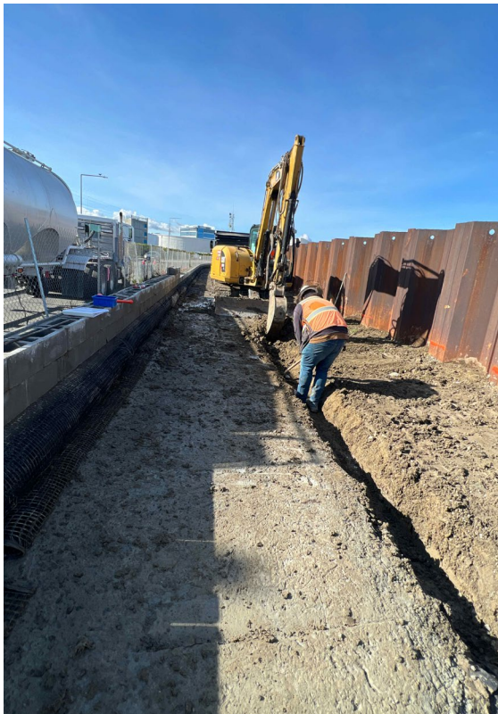
Levee retaining wall under construction
